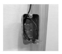
Throughout the following steps, make sure the control cable is kept accessible and protected from damage. It will be needed later to connect the control.
