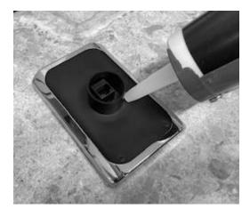
**Step 4:** Connect cable to the control. Ensure that there is a firm connection. Insert the control's tube into the mounting hole and firmly press the control against the wall. Level the control and tape it securely in place [painters tape generally works well] and leave in place until the silicone has cured completely.
